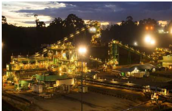
Washing Plant : 525 tph (max: 550 tph)
